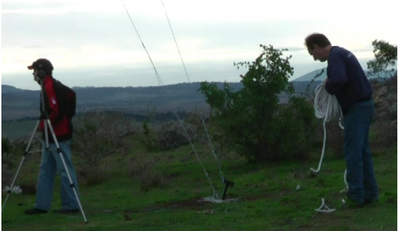
Matthew Cocks and Barry Agg clean up after the job. The antenna is now securely in place.
